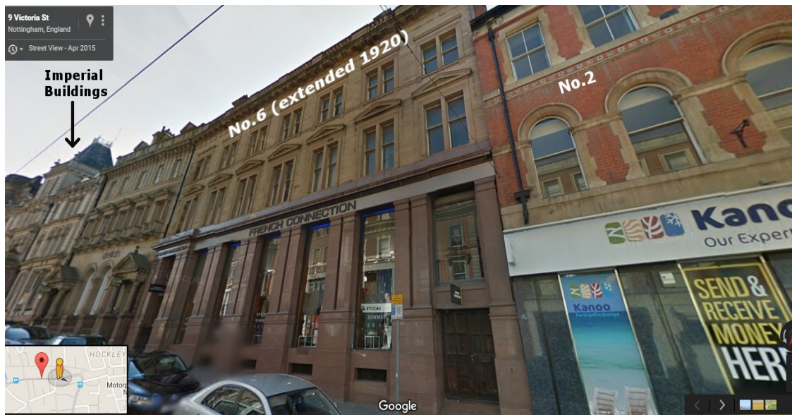
[BB2]. Victoria Street in 2015. Note No.6 has been seamlessly extended into No.4, demolishing it (in 1920) (count the extra columns). Buildings either side have remained unchanged
